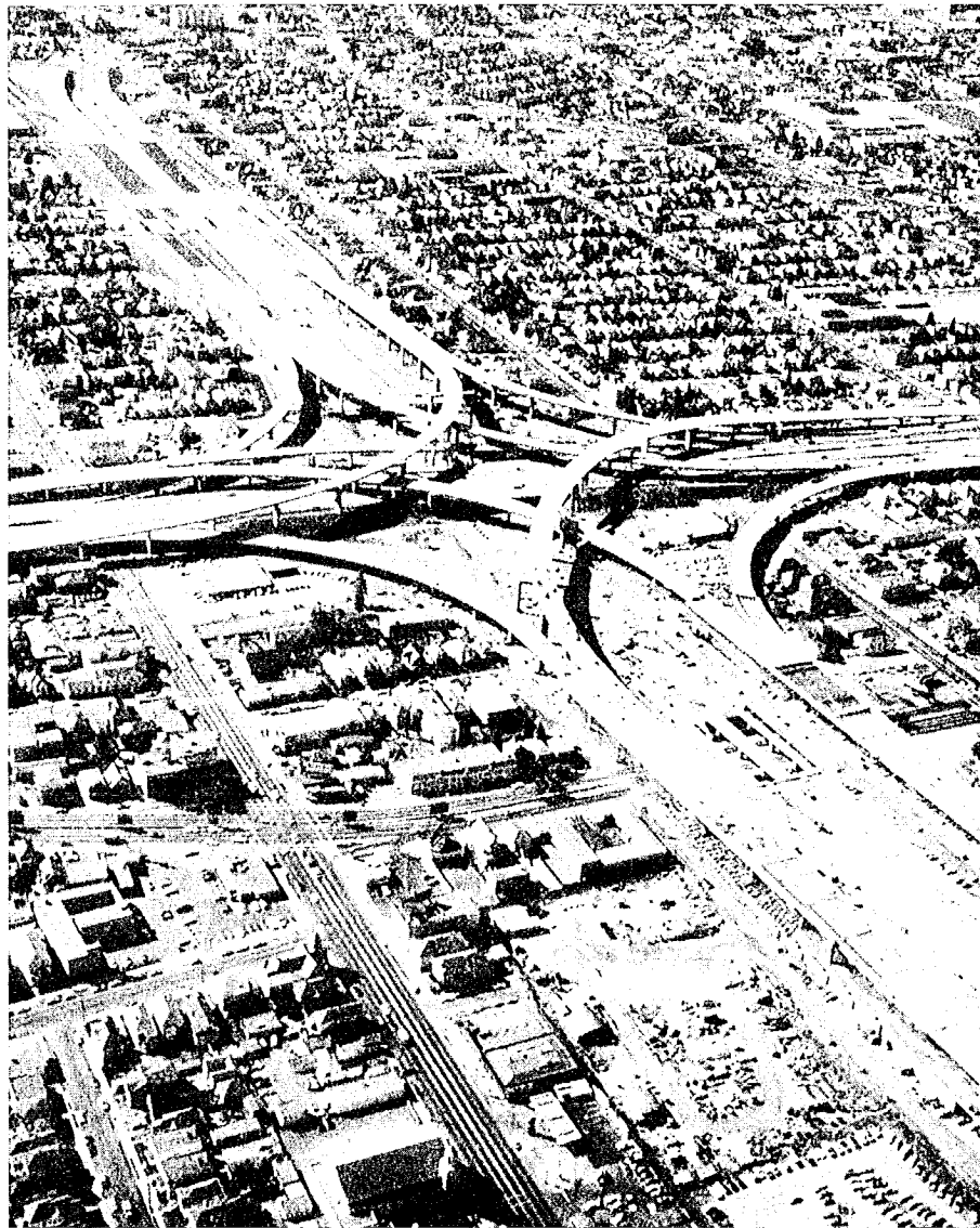
FIGURE 1.5. The I-580/I-980 interchange under construction in West Oakland, California. From Department of Public Works, Annual Report, 1968-1969 (State of California, 1969), 73.
