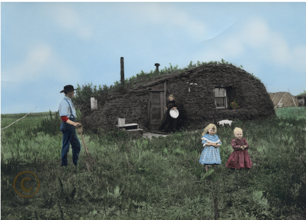
FIGURE 6. John and Marget Bakken sod house, Milton, North Dakota, circa 1895. Photograph by Fred Hultstrund; courtesy of the Fred Hultstrund History in Pictures Collection, North Dakota Institute for Regional Studies—North Dakota State University.
