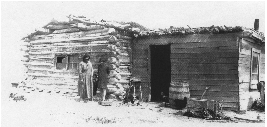
FIGURE 4. Guy Black Hawk home, Fort Berthold Industrial Survey, circa 1922–29. Courtesy of the National Archives and Records Administration, Kansas City, Missouri.
