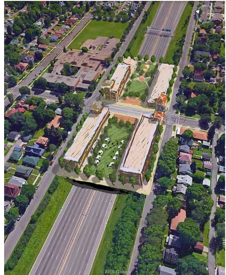
Artist rendition of smaller version of the Rondo land bridge Credit: ReconnectRondo.org
